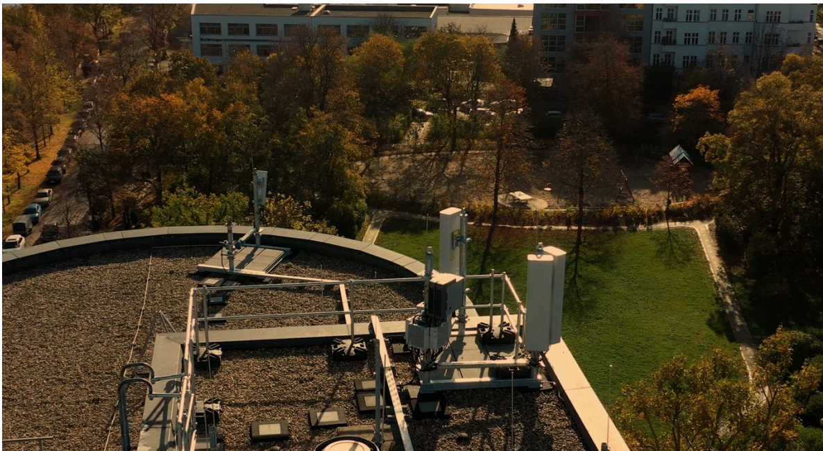
Figure 2-16 5G Radio Units on top of the FOKUS building
