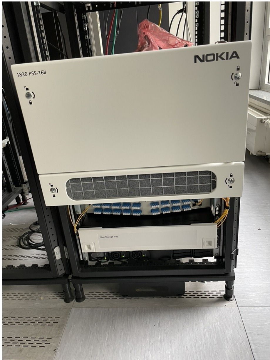
Figure 2-8 Remote DWDM Node “Fokus-2” at FOKUS project data center
