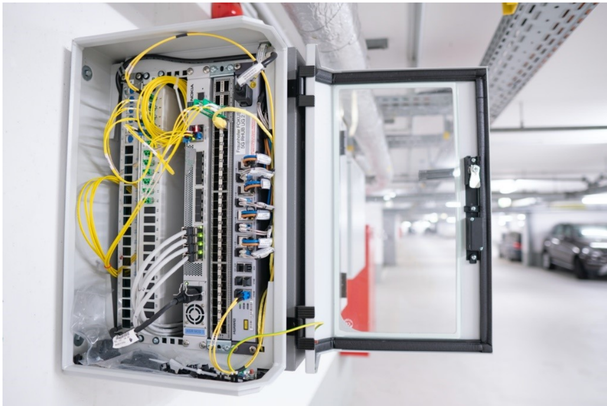
Figure 2-23 Leaf-switch, Huawei Radio Hub and Nokia Radio Hub deployed at the FOKUS parking deck
