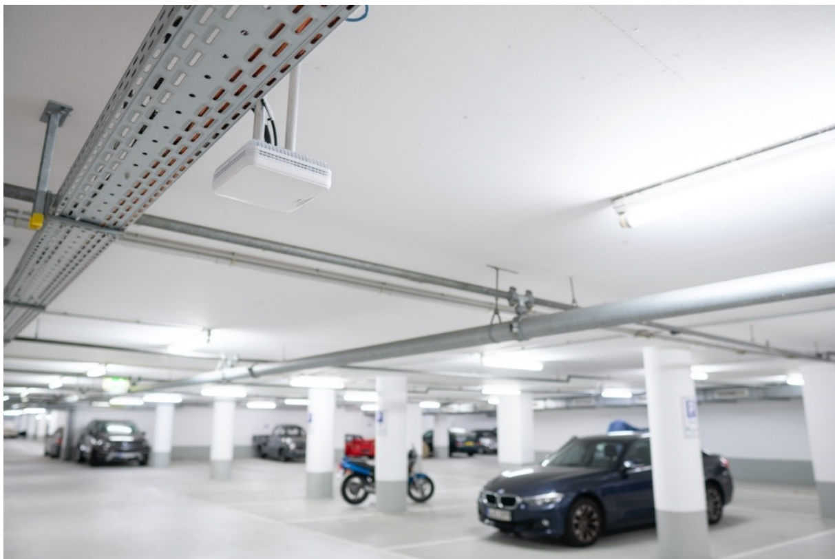
Figure 2-22 Remote Radio Head deployed at the FOKUS parking deck
