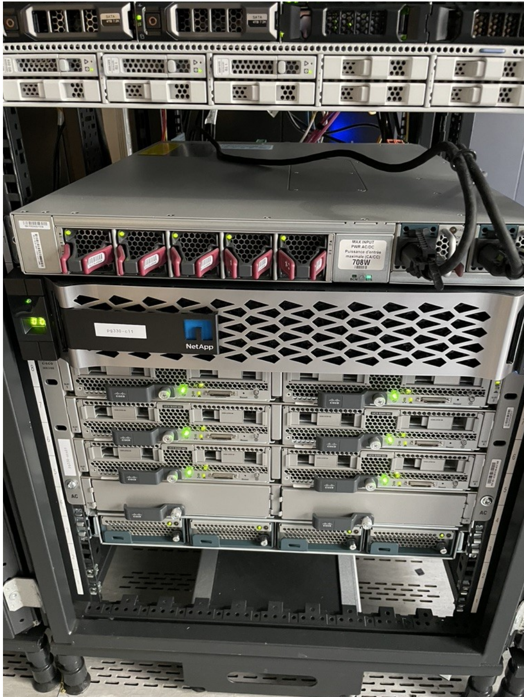
Figure 2-6 Compute and Storage Cluster (Cisco UCS & NetApp) at FOKUS project data center
