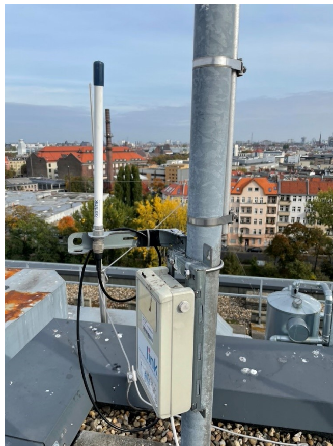
Figure 2-18 LORA access point on the FOKUS roof
