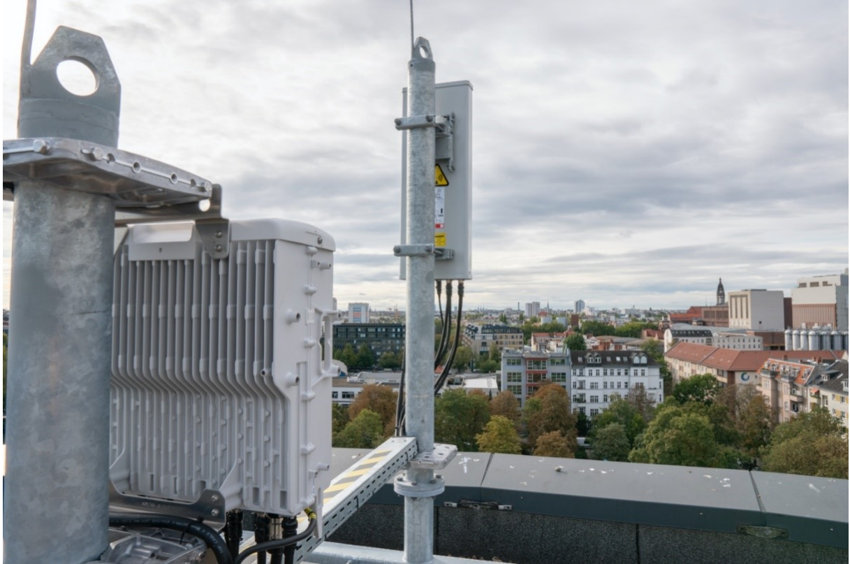
Figure 2-17 Nokia Radio Unit and Sector-Antenna on the FOKUS roof
