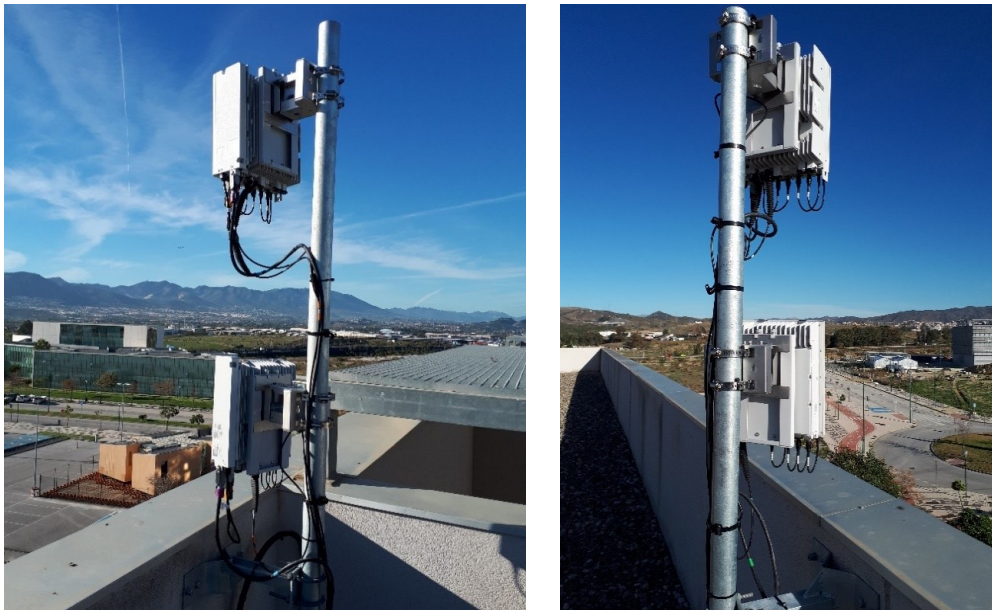
Figure 22: Nokia 5G and 4G micro RRH in Ada Byron building rooftop
