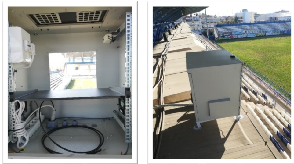
Figure 8: Egaleo Site Cabinets for edge equipment
