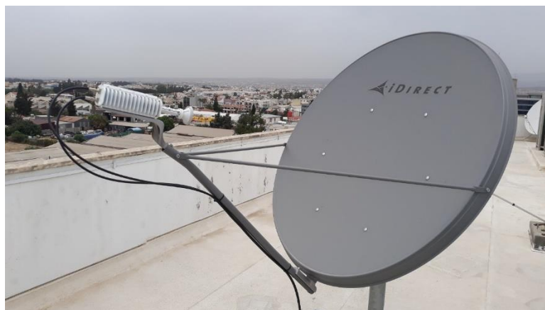
Figure 9. Fixed satellite antenna installed to backhaul the 5G hotspot
