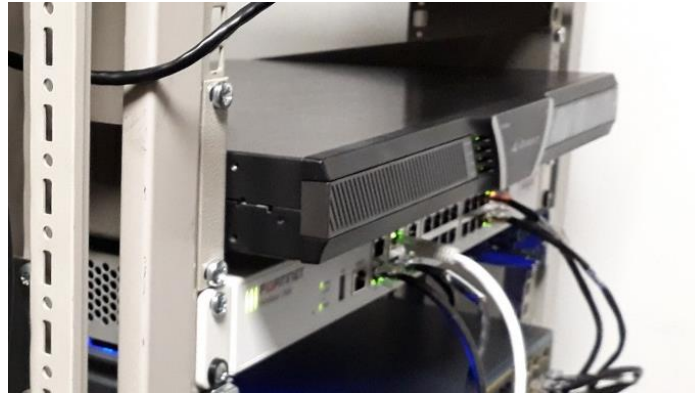
Figure 8. iDirect X7 satellite terminal installed at 5GENESIS platform
