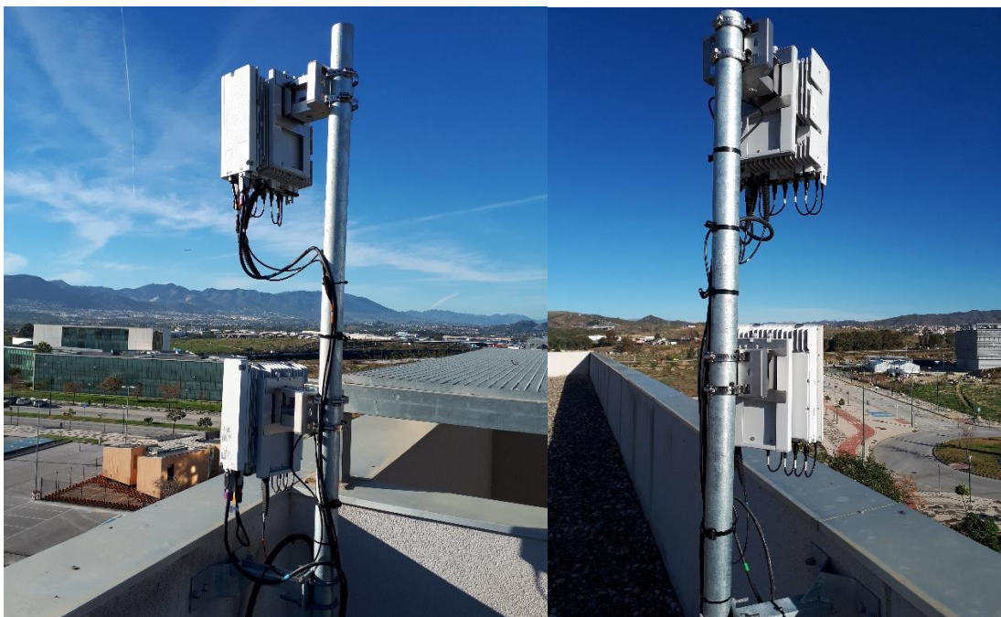
Figure 18: Nokia 5G and 4G micro RRH in Ada Byron building rooftop
