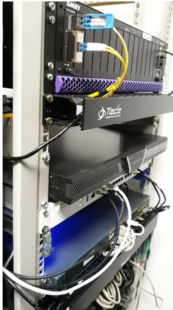
Figure 7-2 Limassol platform setup equipment
